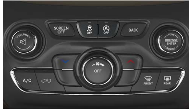
Manual Temperature Faceplate Controls
