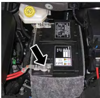
Positive Battery Post
