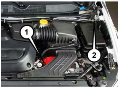
Positive Battery Post
