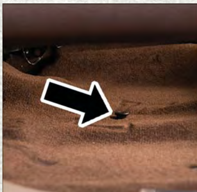
Floor Fastener Location
