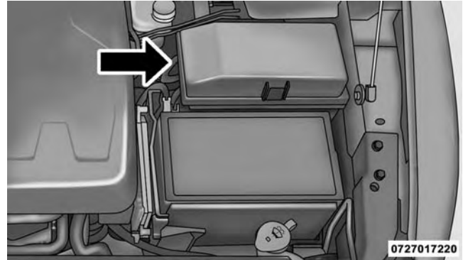
Power Distribution Center
