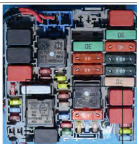
F30 Fuse 20 Amp Yellow Power Outlet – Center Console F84 Fuse 20 Amp Yellow Cigar Lighter/Power Outlet Instrument Panel
