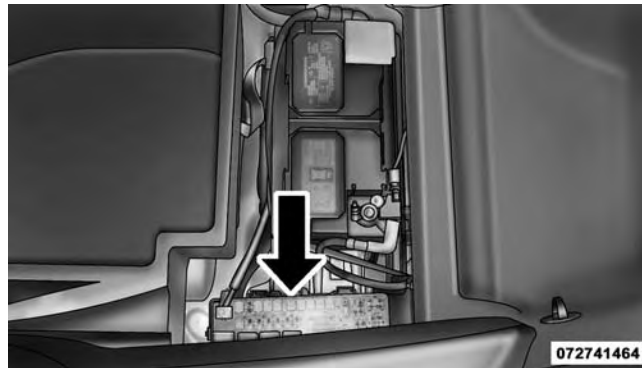
Rear Power Distribution Center
