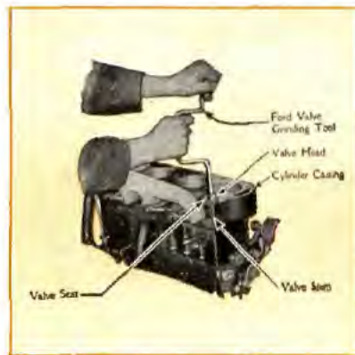
Method of grinding valve. (Cut No. 5)
